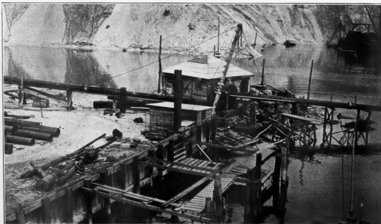
Booster Pump Between Dredge and Screening Plant
